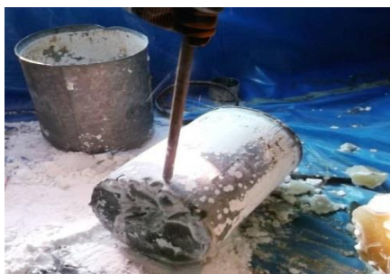
Fig 3. Dismantling of DSRS Container
