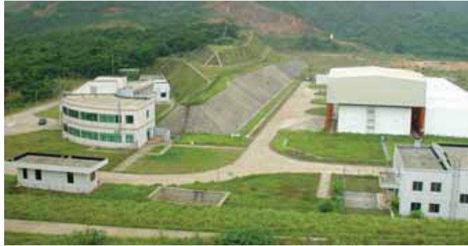
Figure3.2-3 The picture of the Beilong LILW Disposal Site (Credit of Guangdong Nuclear Engineering Cooperation)
