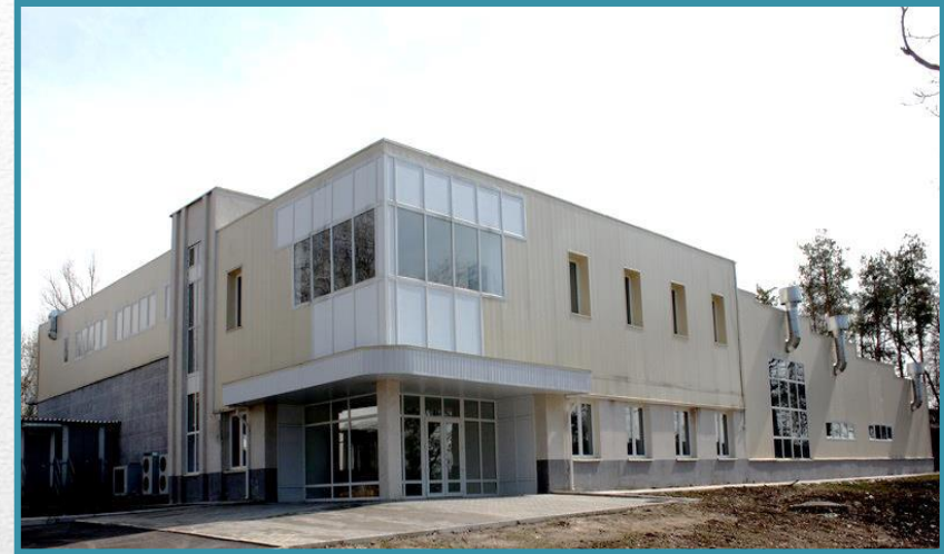
Building of Radiation Sterilization with ILU-10 Accelerator
