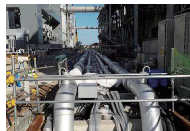
Land-side impermeable walls utilizing the frozen-soil method
