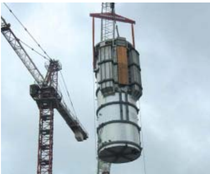
The reactor pool being lowered into position
