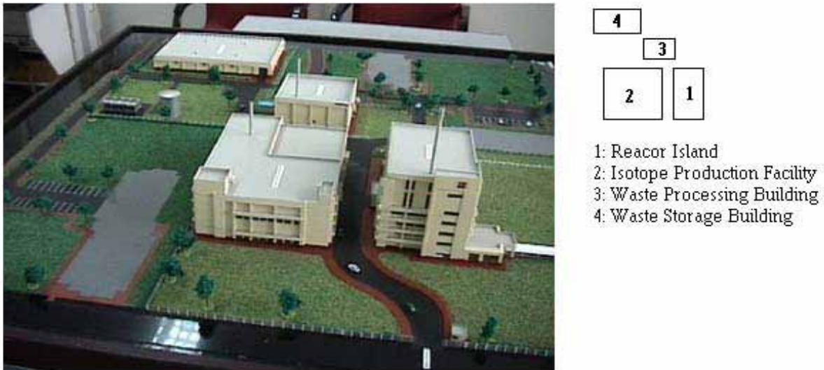
Fig.2 The three main facilities of Ongkharak Nuclear Research Center (ONRC)
