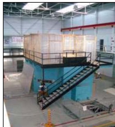
Preliminary dismantling tent (Jan 2009)
