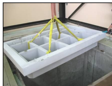
Figure 2: Installation of pit guide frame
