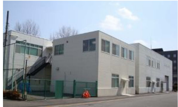
Figure 1 Fuji Electric Systems Calibration facility building
