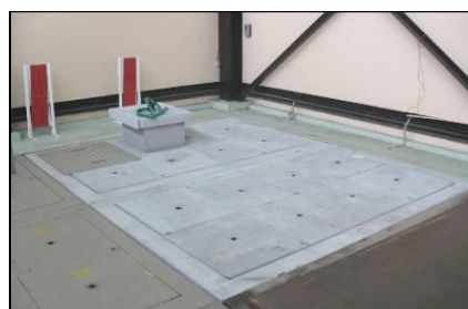
Figure 3: Fully installed pits
