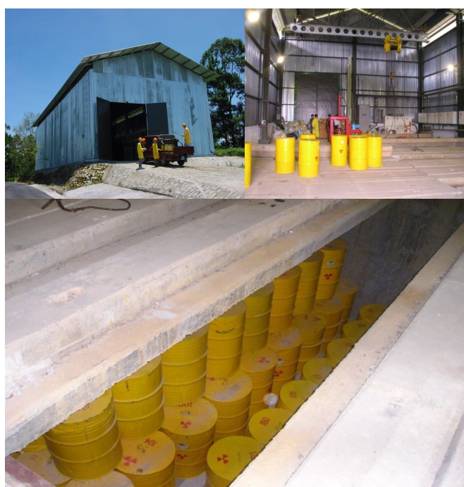
Fig 1. On-site storage at DNRR
