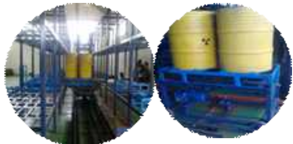
Testing and Commissioning of ASRS
