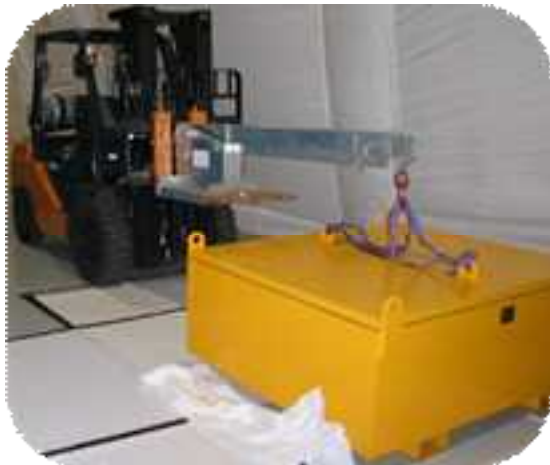
Figure 2: Lifting 50mm steel box
