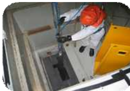
Figure 1: Lifting graphite from reactor core
