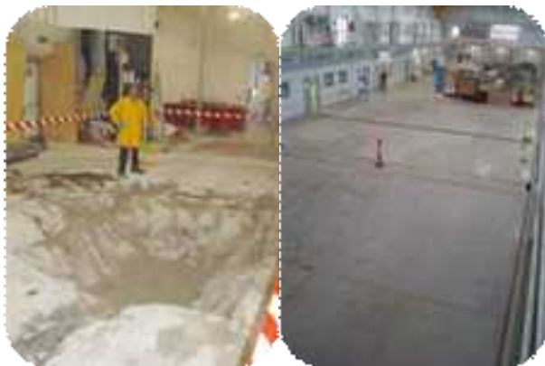
Figure 6: Excavated and remediated floor
