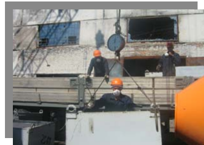
Fig3: Loading of containers with solid radioactive wastes into cargo truck
