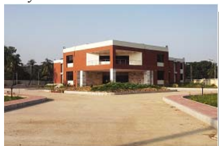
Fig1: Two storied laboratory building
