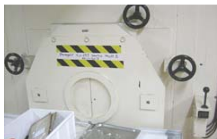
Fig8: Hot Cell posting port to be fitted with a safety interlock.
