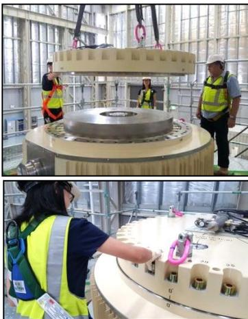
**Figure6: (a) Lowering of the secondary lid over the primary lid of the TN81. (b) Positioning the bolts for securing the secondary lid.**
