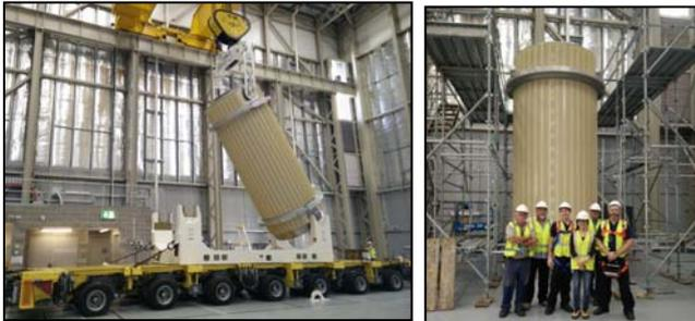
**Figure5: (a) Tilting and lifting of the TN81 from the transport frame. (b) Handling team posing in front of the vertically positioned TN81.**
