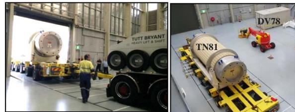
Figure4: (a) TN81 arriving into the IWS on the back of the transport trailer. (b) DV 78 and TN81 inside the IWS.
