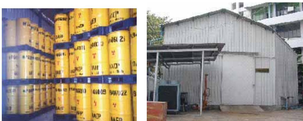
Fig. 3.8-6 Waste Storage Facility for RI waste at OAP
