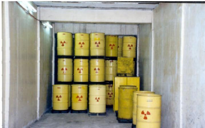
Figure 3.7-3 Interim Storage - Engineered Trench
