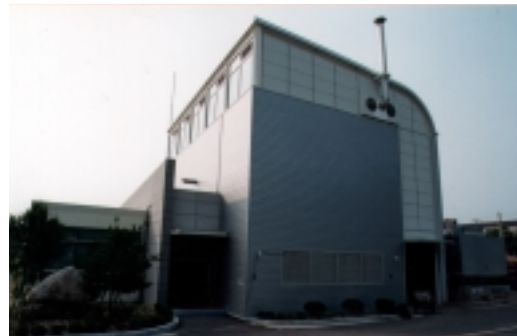
The exterior view of Vitrification Facility for LILW in Korea
