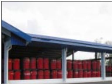
2,400 drums of oil sludge have already gathered in the storage facility of MINT.
