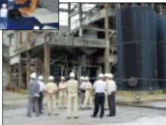
Site visit to the plant undergoing dismantling
