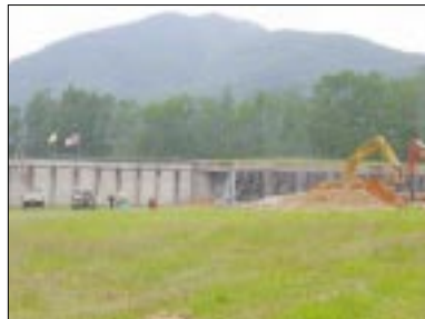
The reconstruction of LTSF (Long Term Storage Facility) has begun.
