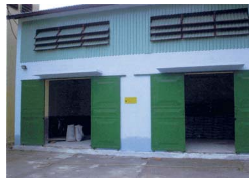
The radwaste treatment house
