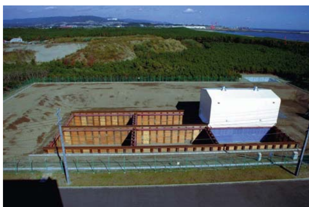
Figure 1 Waste Disposal Facility in JAERI
