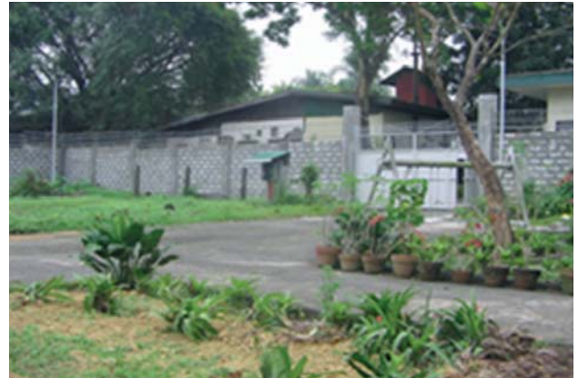
Upgrading of Perimeter Fence of the Facility
