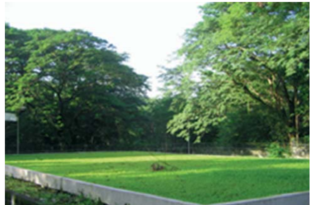
Top View of Engineered Trenches
