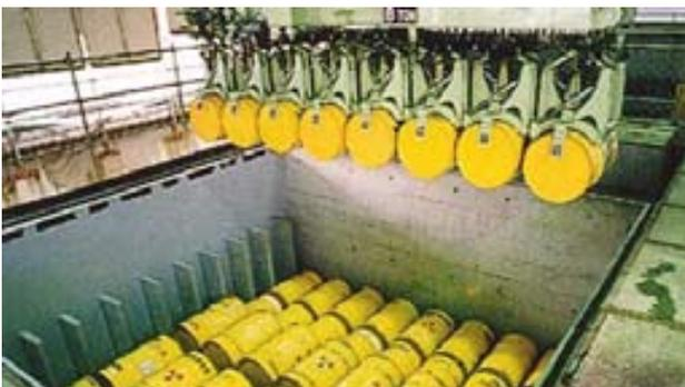
**Stacking Drums Waste packages are stacked inside the disposal facility.**
