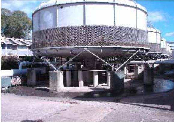
**Fig 9:** Secondary cooling system towers
