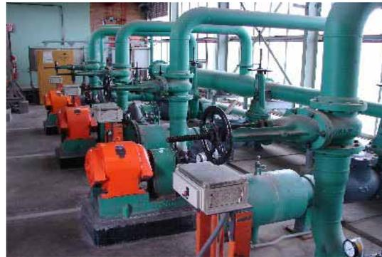
**Fig 8:** Secondary water cooling system pumps to be demolished
