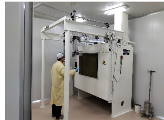
RI production facilities
