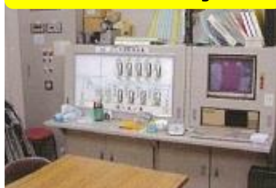
Radiation monitor room for ventilation and drainage tank
